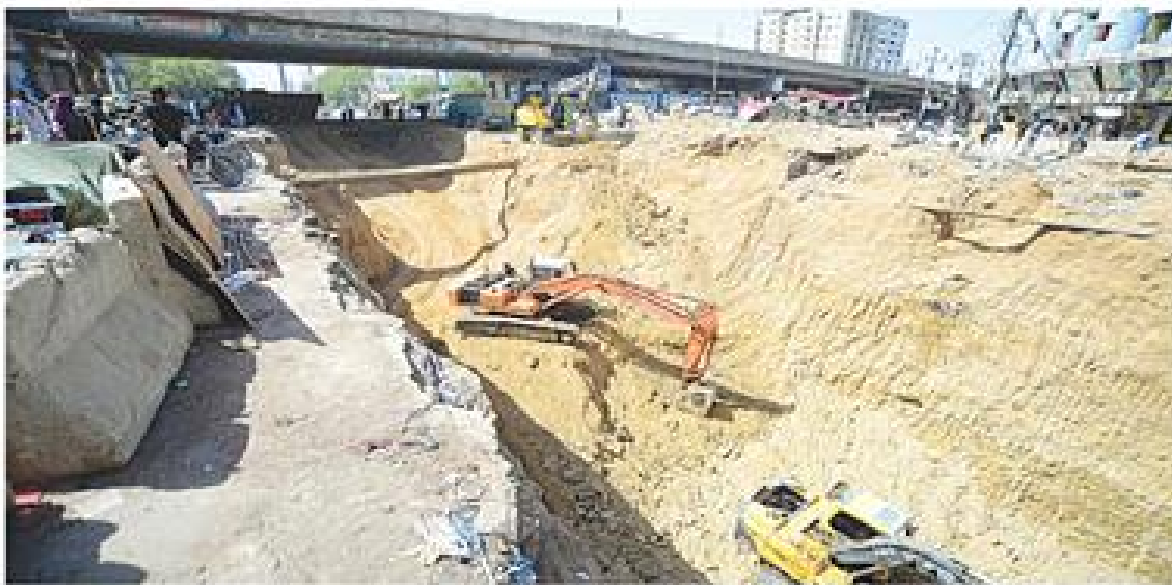
EXCAVATORS work at the construction site of the Karimabad underpass. — PPI
