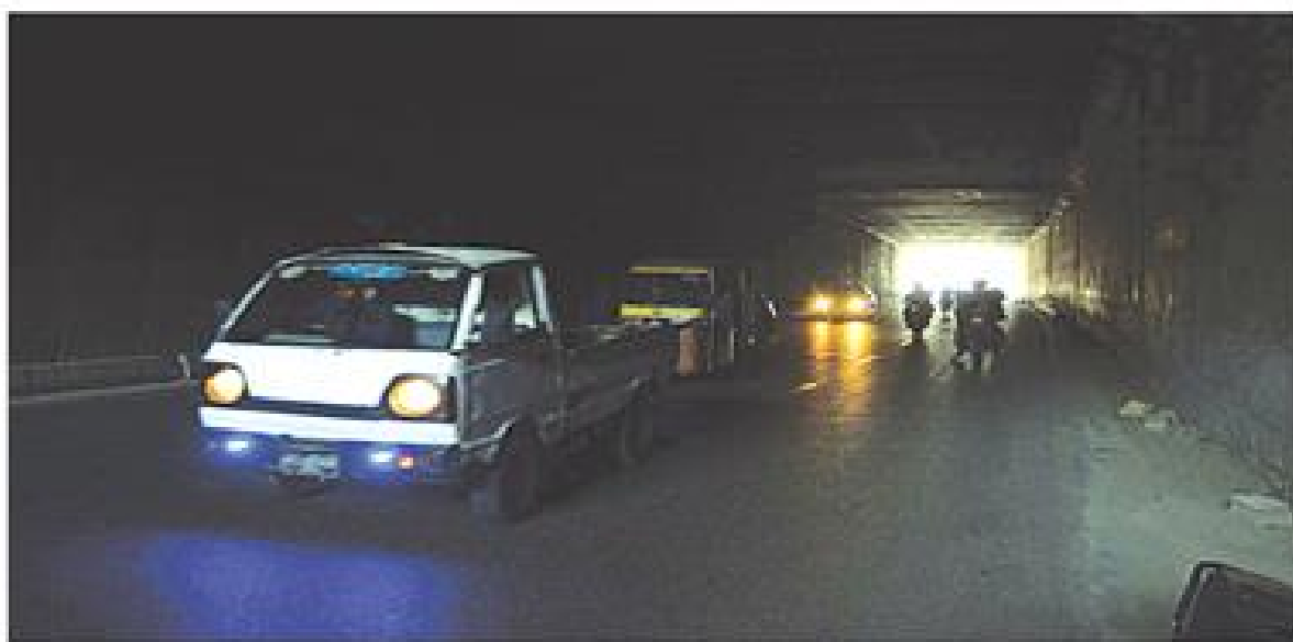
MOTORISTS turn on their headlights during daytime as they pass through the unlit Nazimabad underpass, on Wednesday. The subterranean passage is dangerous and accident-prone due to a lack of illumination. —FPF
