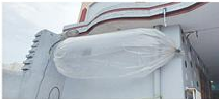
A GAS-filled plastic bag installed outside a house on the outskirts of Peshawar. — Dawn
