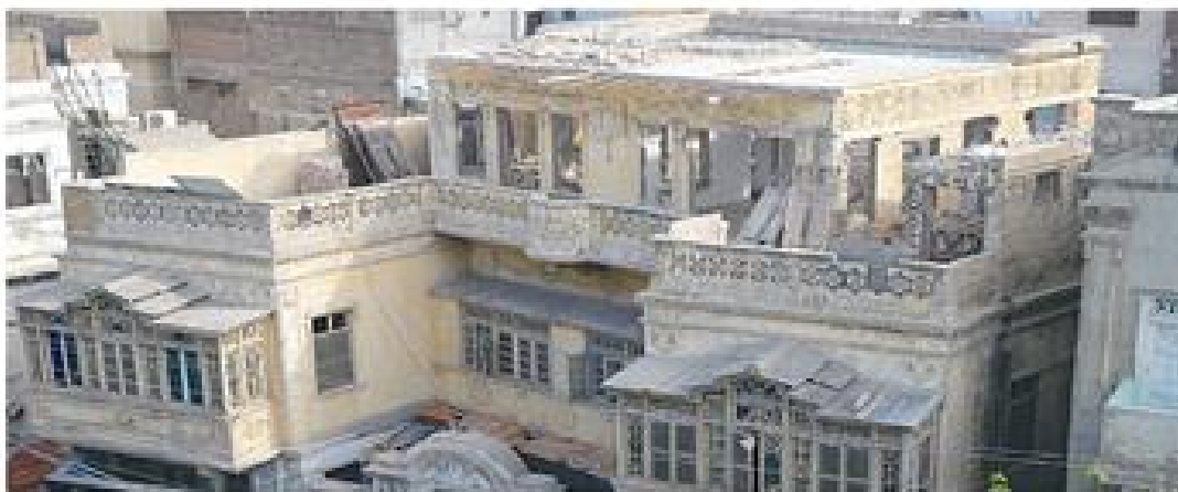
THE second floor of the 1938 heritage structure undergoing demolition in Hyderabad, on Monday.—Photo by Umair Ali
