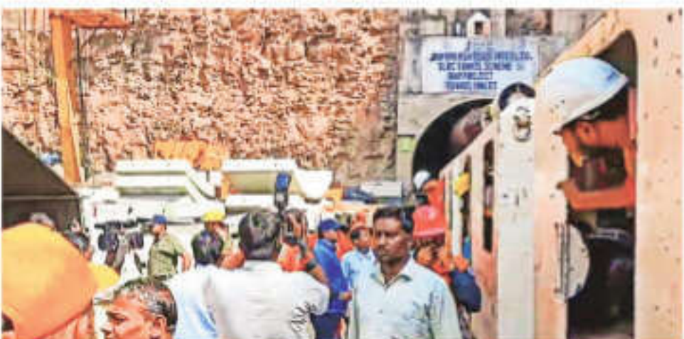
Rescue operation underway to trace the workers trapped inside the tunnel in Nagarkurnool, Wednesday. PTI
