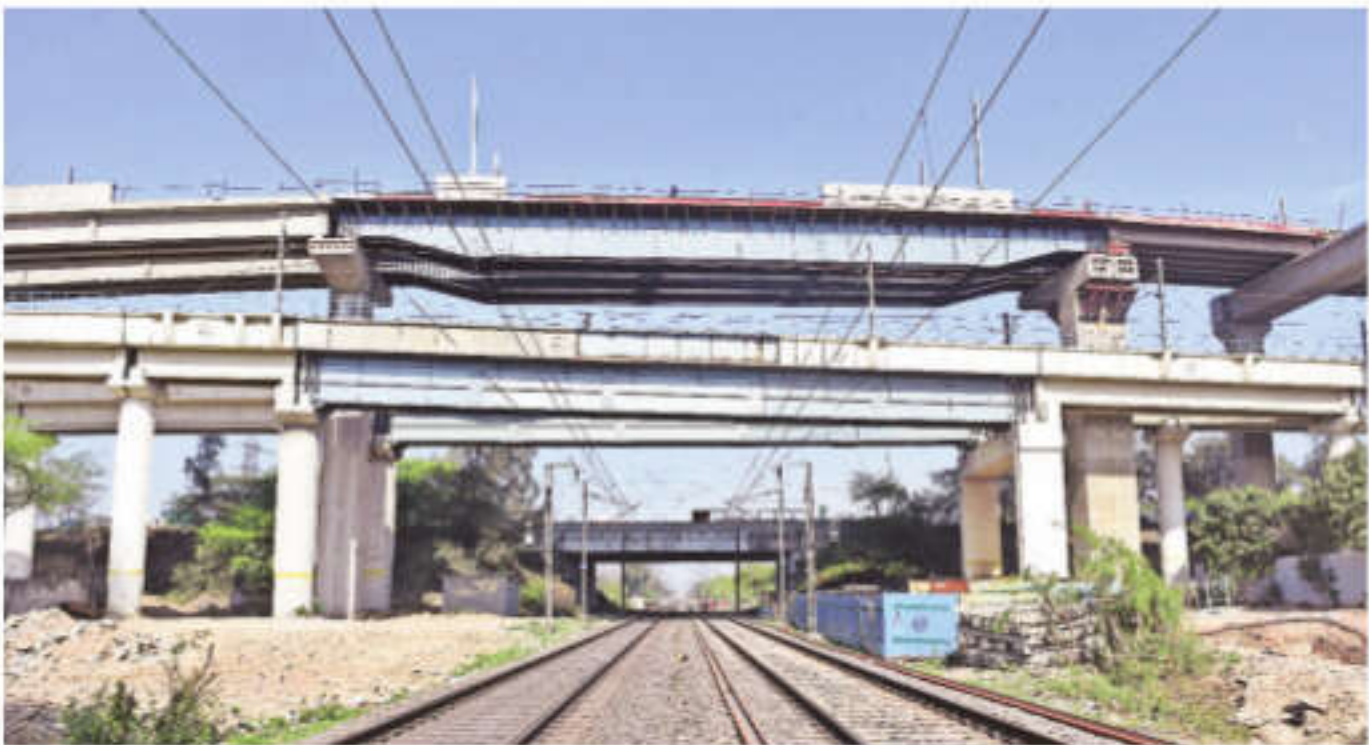
The steel span was constructed over the operational Yellow Line, ensuring minimal disruption to Metro services and live railway line. Credit: Express
