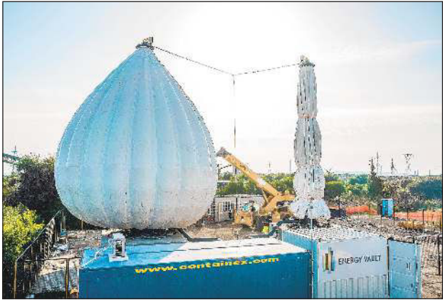
WATER TREES are filled in Sardinia, Italy, last year. One 39-foot-tall tank can hold enough water to release about 800 gallons a minute for three hours.
