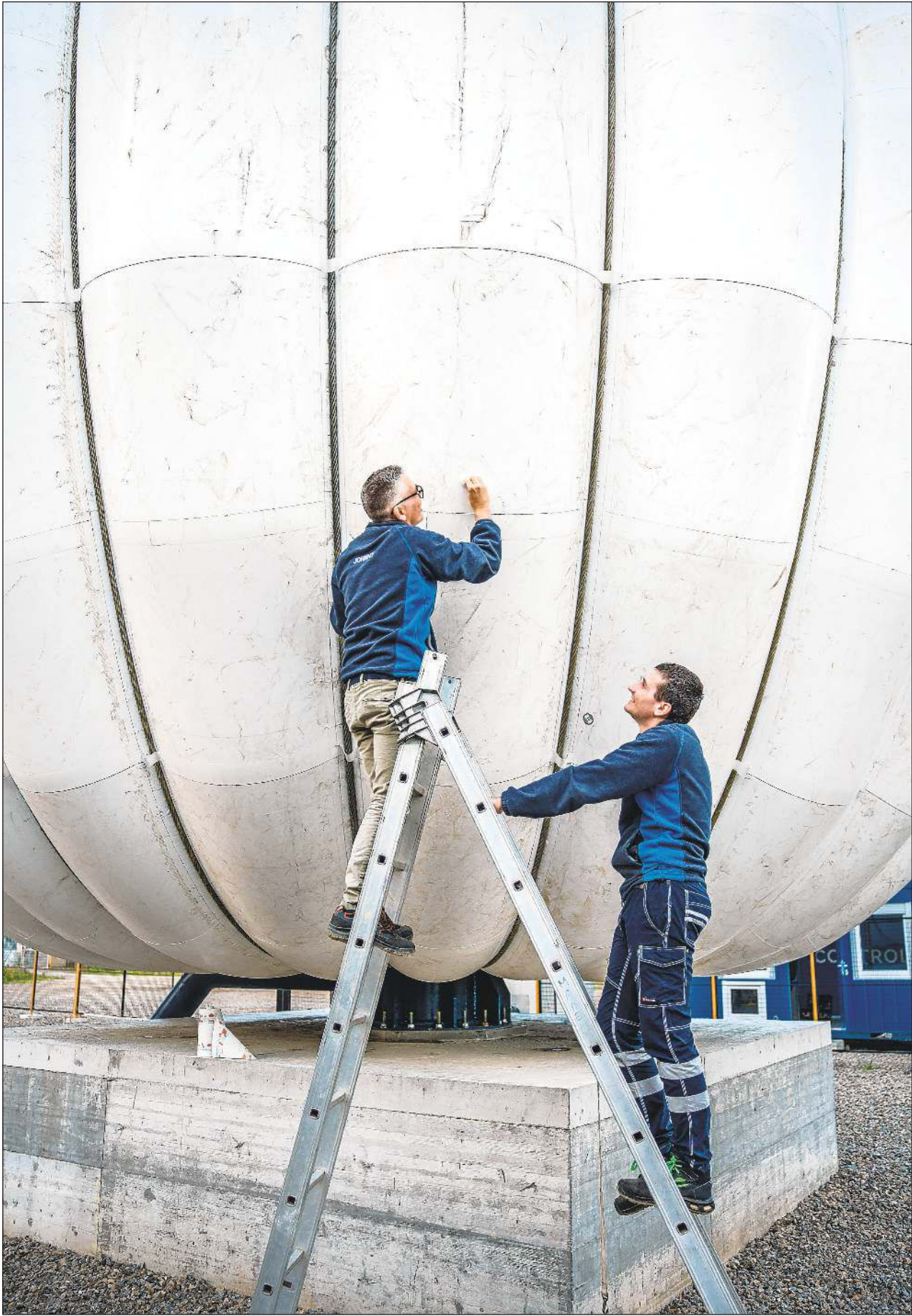
WORKERS in Sardinia, Italy, last year inspect the membrane that holds water, which is designed to last more than 20 years. A concept envisions installing 40 or 50 of them in Pacific Palisades as areas are rebuilt.
