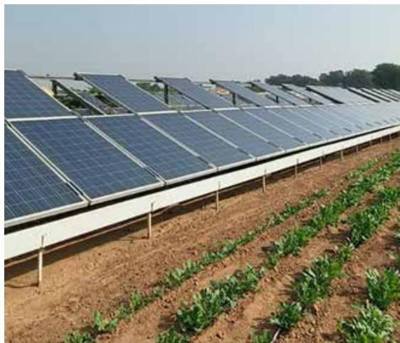
FIGURE 6.2 105 kW APV at ICAR-CAZRI, Jodhpur, Rajasthan
