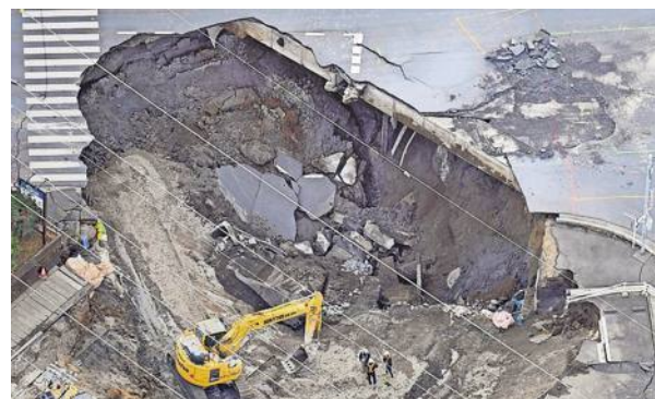
The sinkhole was caused by sewage leaking from a pipe, softening the soil
