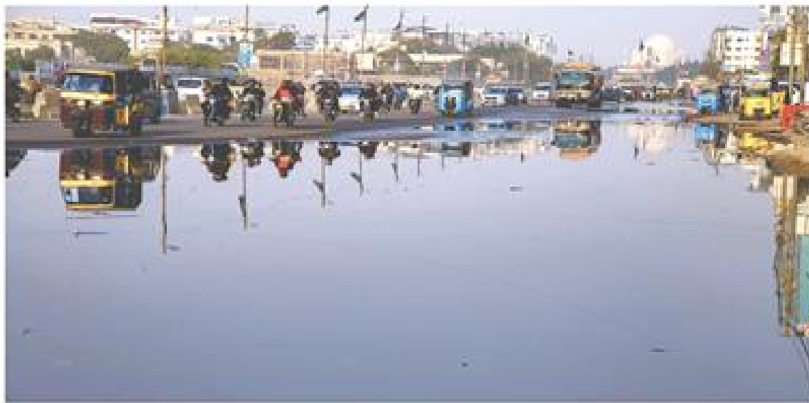
TRAFFIC moves at a snail's pace on the M.A. Jinnah Road as the thoroughfare is submerged by sewage, on Sunday — PPI
