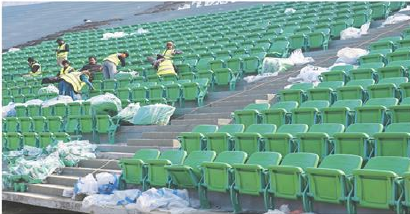
NEW chairs are being affixed at Gaddafi Stadium as a part of remodeling and upgrade. — White Star
