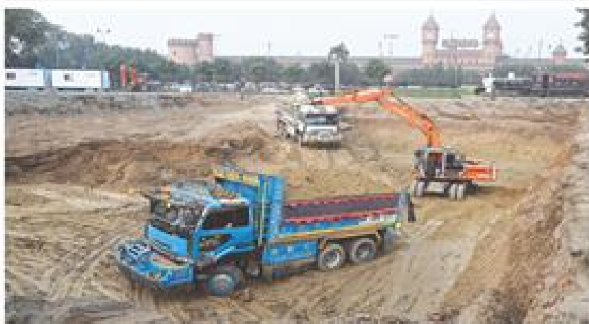
THE construction of fifth water tank in front of railway station underway. — White Star
