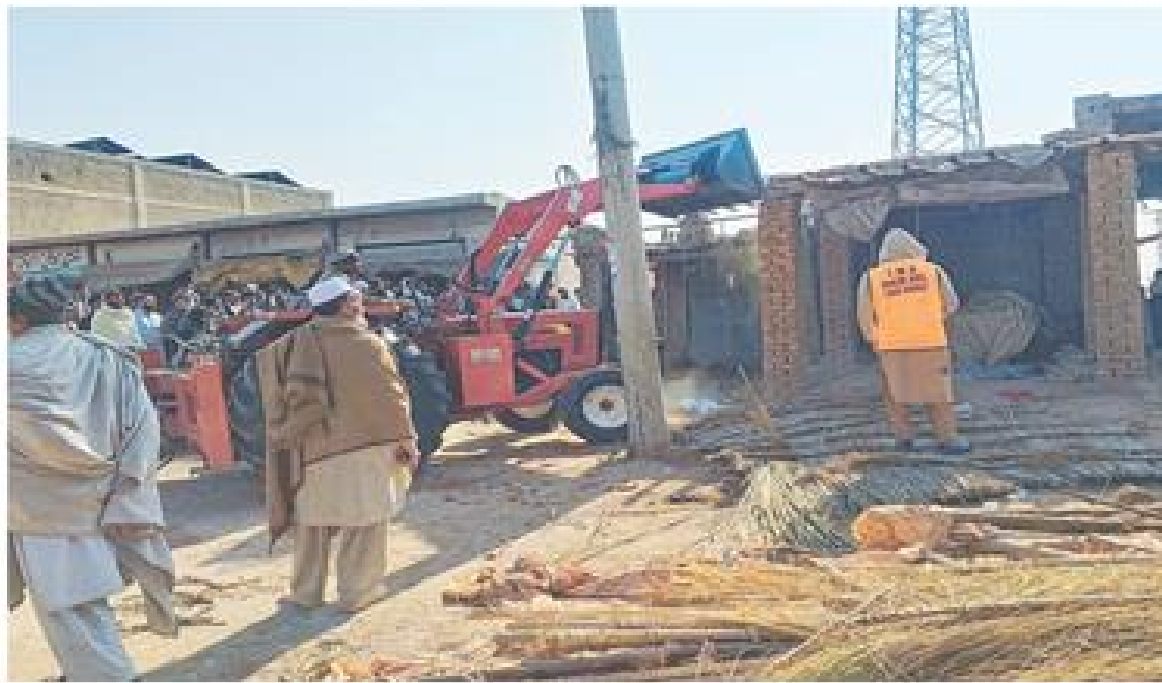
THE TMA staff demolishes illegal structure during an anti-encroachment drive in Ghazikhet Bazar, Lakki Marwat on Sunday. — Dawn
