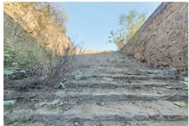
THE stone-cased passage was used by horses to directly access water during wars around Rohtas Fort.
