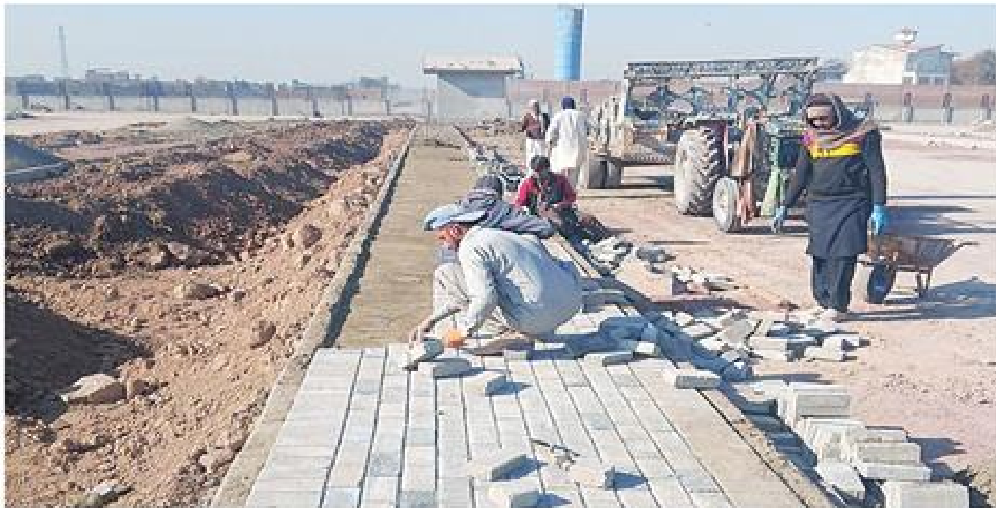
WORKERS lay concrete tiles on a pavement at new bus terminal in Sander Garhi, Peshawar, on Monday. — Wafa Sitar
