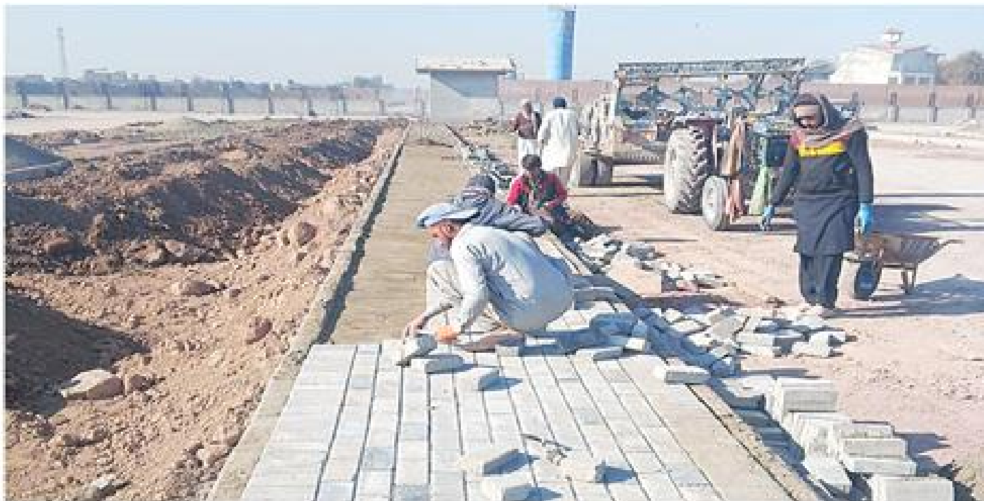
WORKERS fix cement tiles on a pavement at new bus terminal in Sardar Garhi, Peshawar, on Monday. — White Star
