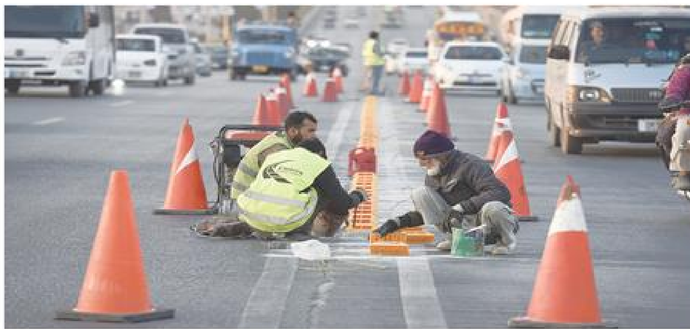
WORKERS install cat's eye reflectors on Islamabad Expressway near PWD interchange on Saturday. — Photo by Tarveer Shehzad
