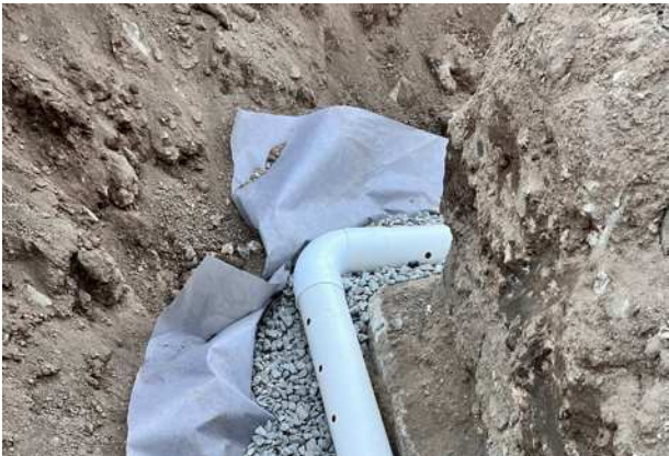
Almost everything about the installation of this 4-inch-diameter perforated drainpipe is wrong. TIM CARTER
