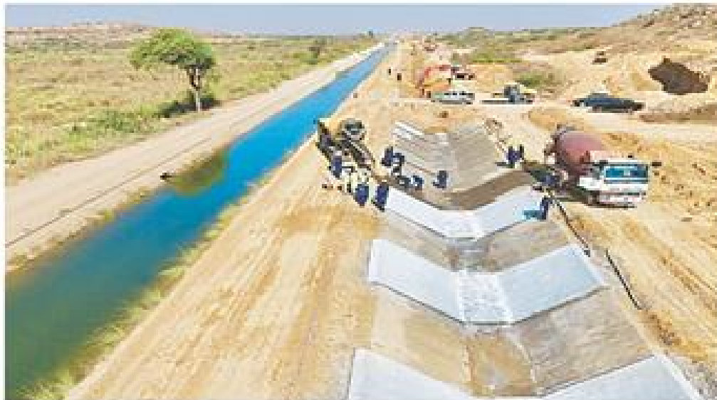
WORK to construct a new canal to bring water from Hub Dam to Karachi is underway. Mayor Murtaza Wahab (right) inspects the progress during a visit to the project site, on Tuesday — Dawn
