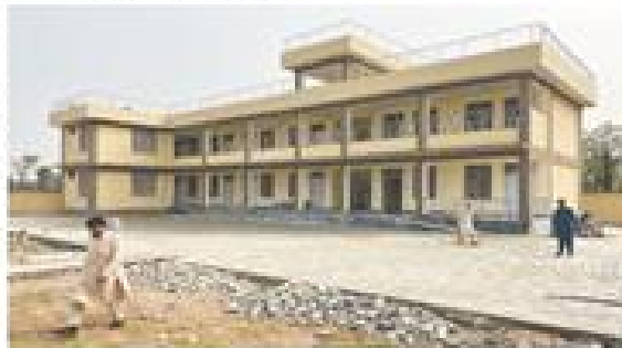
A VIEW of a newly-constructed primary school building in Sipah area of Bannu. —Dawn
