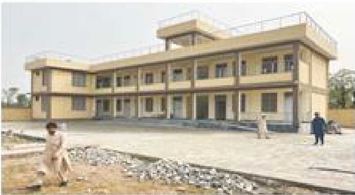
A VIEW of a newly constructed primary school building in Siph area of Bana. — Dawn
