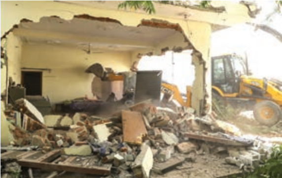
A file picture shows a bulldozer being used to demolish the illegal construction belonging to a person accused of a knife attack on RSS members in Jaipur. — PTI
