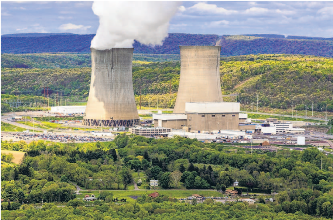
Federal regulators rejected a deal that Amazon had signed with Talen Energy to plug a data center into its Susquehanna nuclear power plant in Pennsylvania, above.
