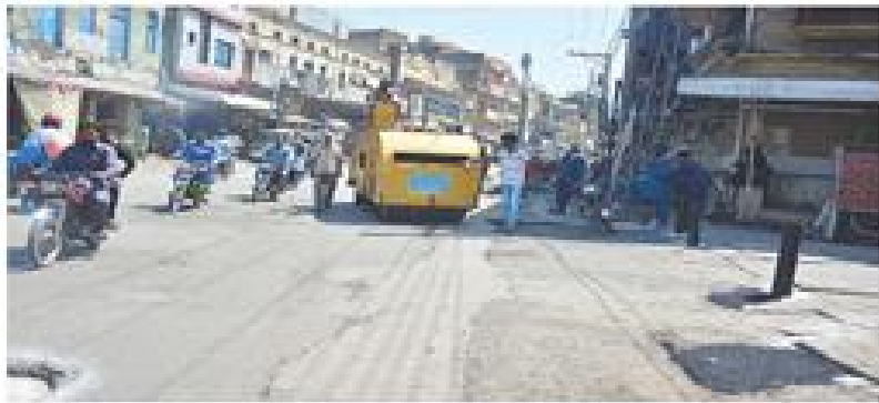
RAWALPINDI Municipal Corporation workers repair the roads that fell on the route of the Ashura procession. —Online
