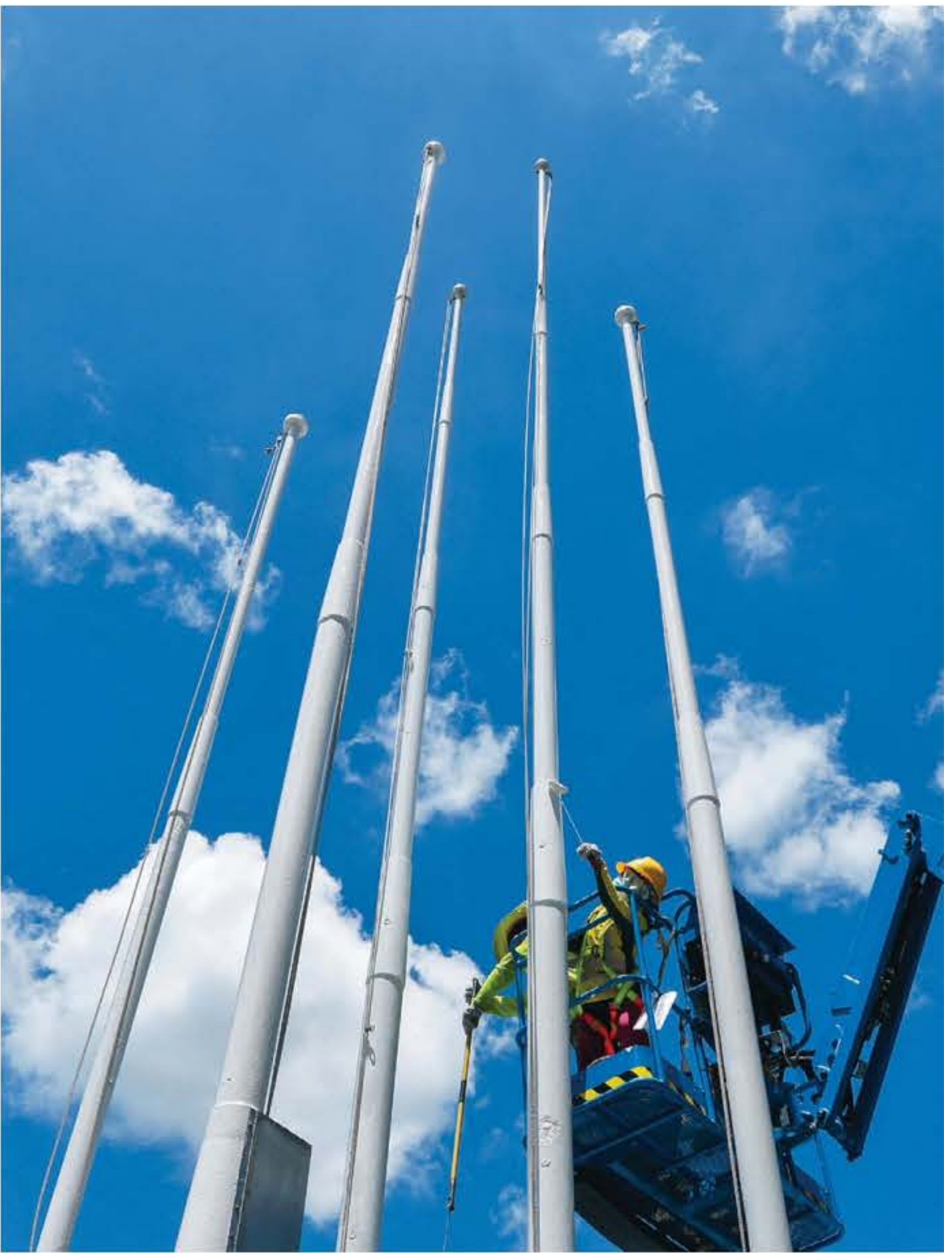
The five flagpoles on the Tsim Sha Tsui waterfront are repainted ahead of National Day. Photo: Elson Li
