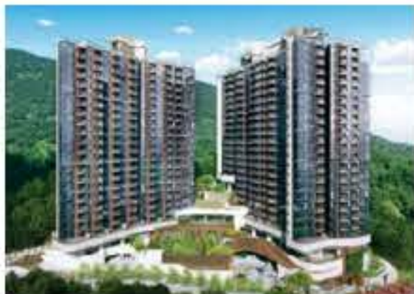
The Uppland comprises two towers with a total of 692 flats.
