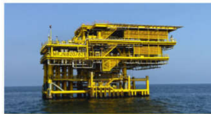
Oil Production Deck Module in Saudi waters
