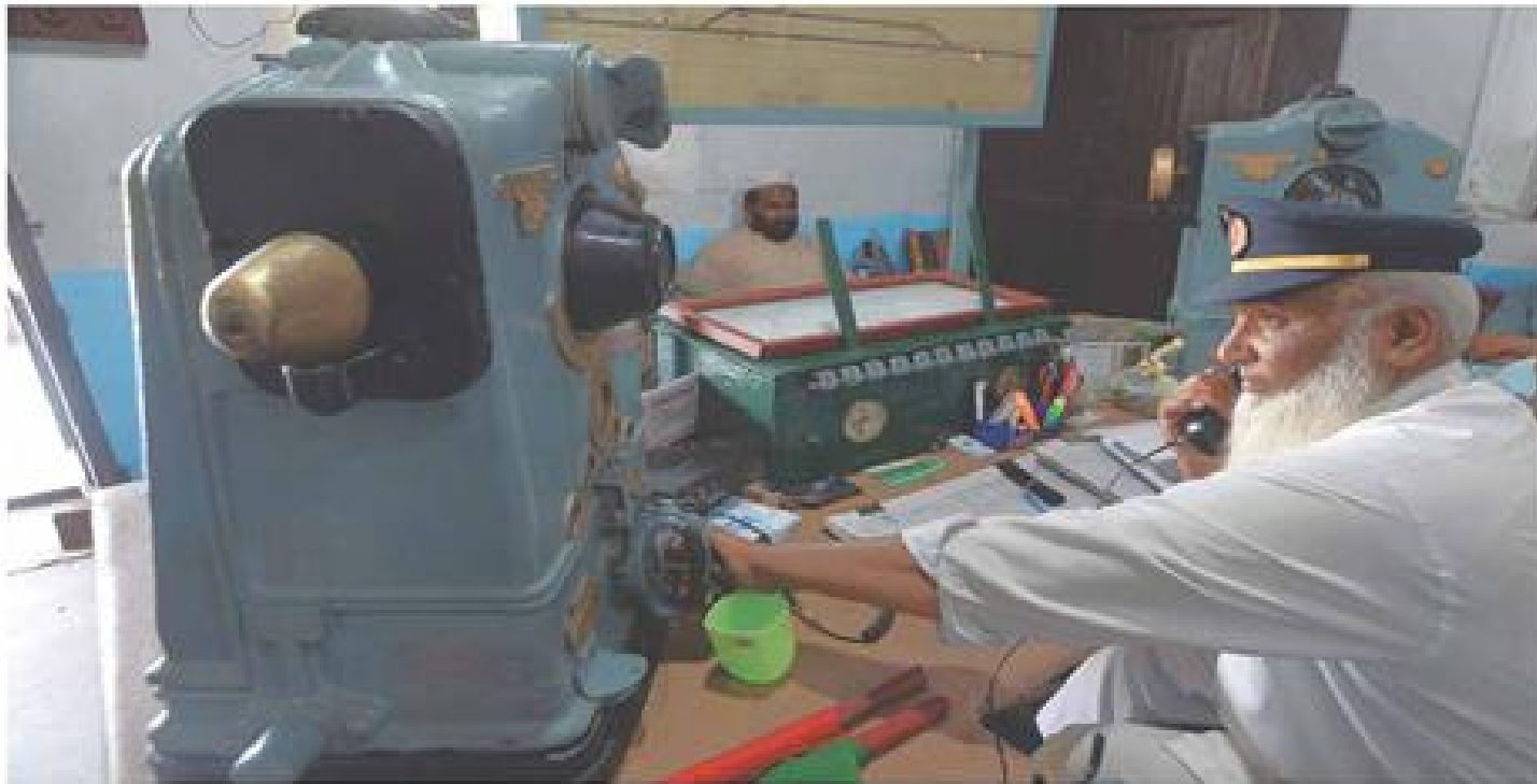
An official uses a tokenless block instrument at Attock Khurd railway station to ensure there is no other train on the track until the next station. The 100% system for use on single track railways has been designed in such a way that the controlling signals will only allow one train to enter the line at any one time. — Wafa Star
