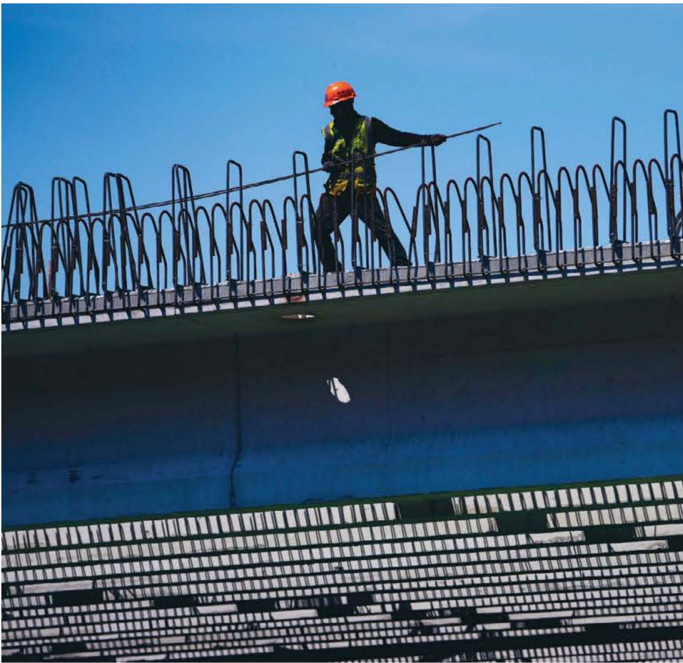
A worker loads a steel cable at a construction site in Beijing yesterday. The global steel wire market was worth about US$69 billion in 2023 and is expected to grow to around US$115 billion
