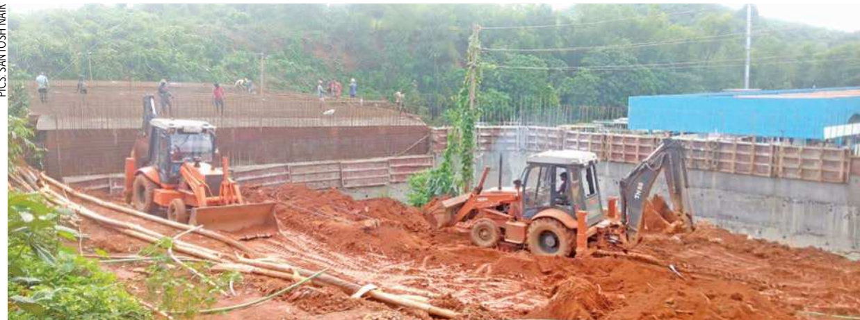
Earth moving machinery undertaking the landfilling work for a ramp to the underpass at the Khandepar-Opa Junction, on Tuesday
