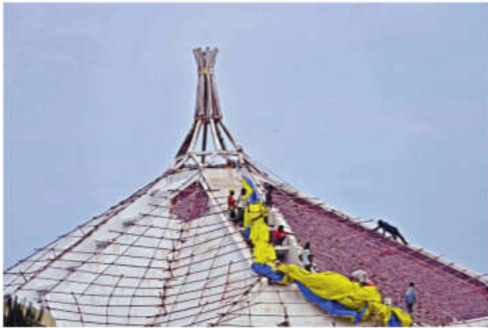
Waterproofing work being carried out at the State Assembly building.
