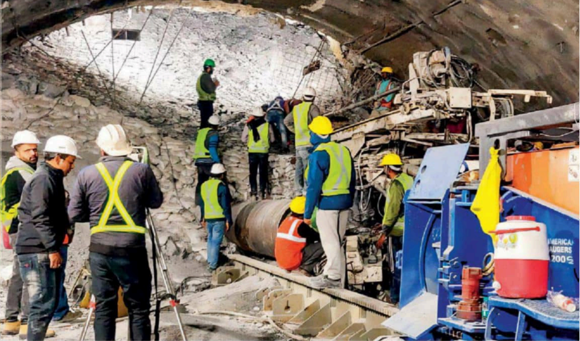
Rescuers in the process of laying a 3-foot-wide pipe through the pile of debris.
