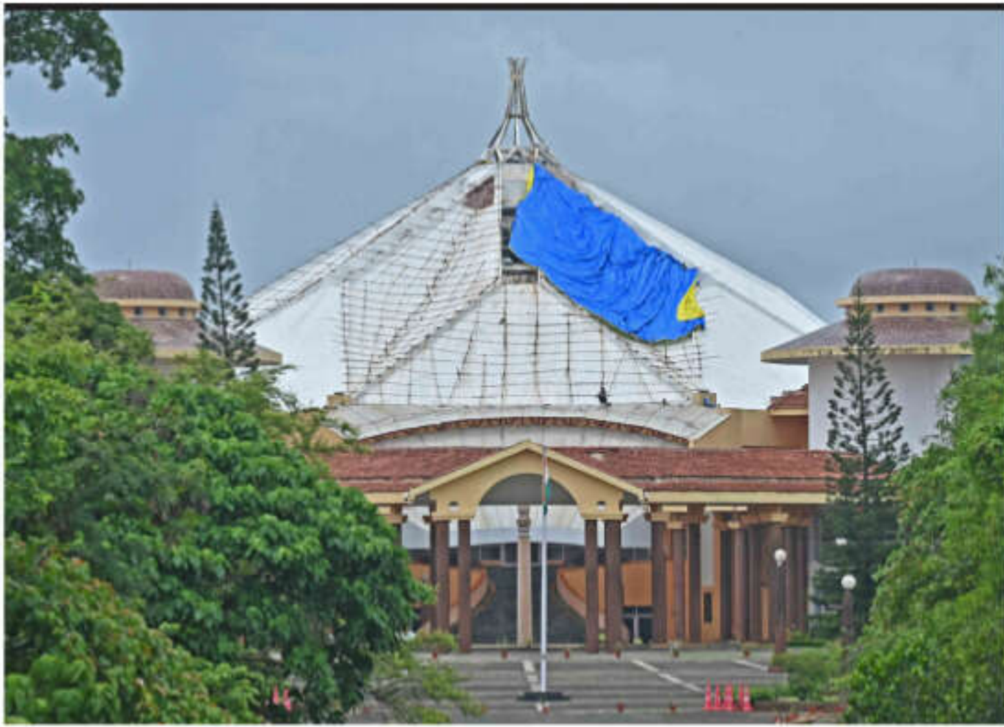
Workers are seen waterproofing the roof of the main dome of the Assembly complex at the start of the monsoon season. Narayan Pissurlenkar
