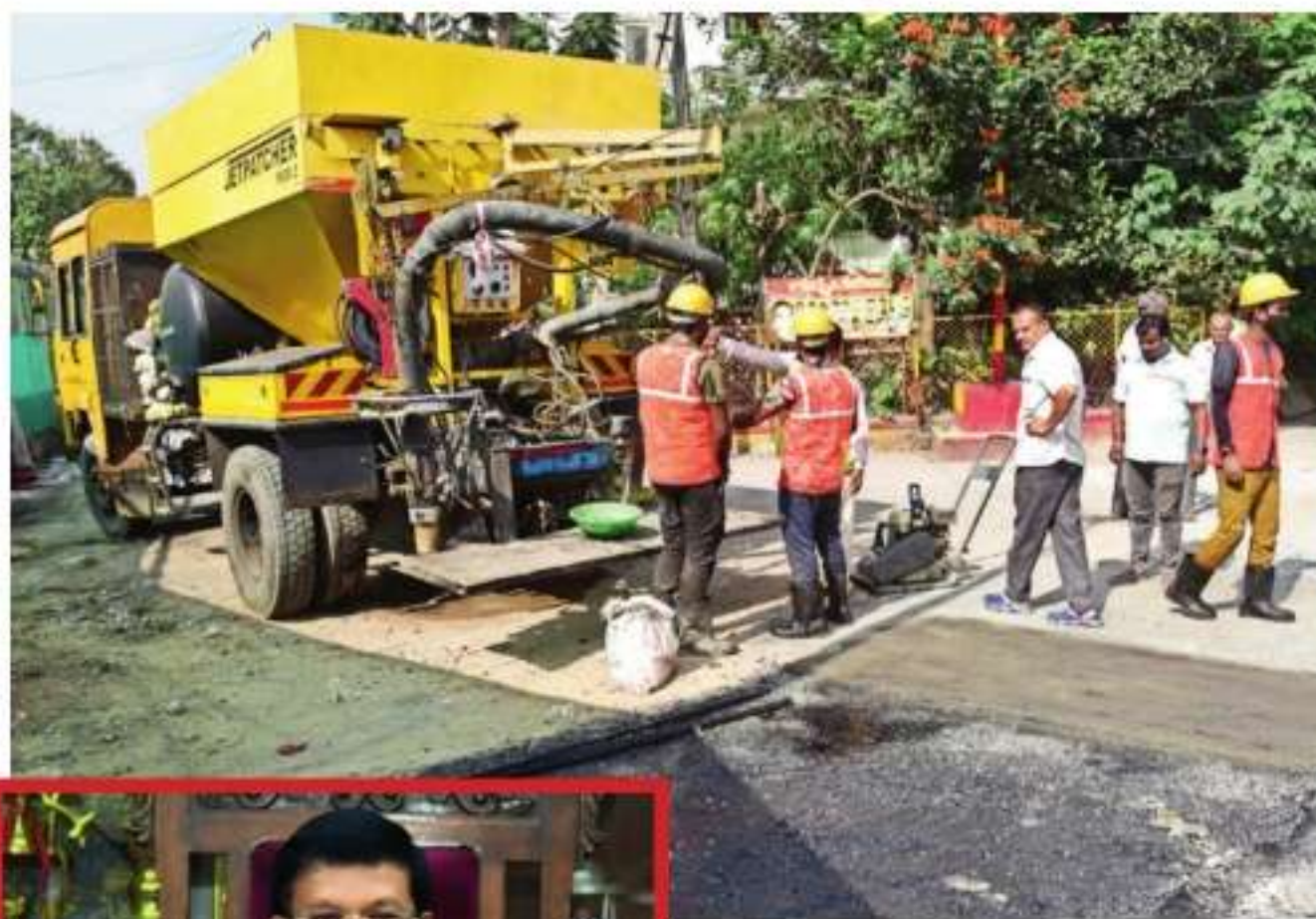
A spray injection road repair equipment, being used to patch a pothole in the city; Inset: Umashankar intends to focus on durable solutions
