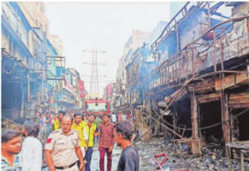
Police and locals near burnt shops after a massive fire broke out in the Shaheen Bagh area, Saturday evening. PTI
