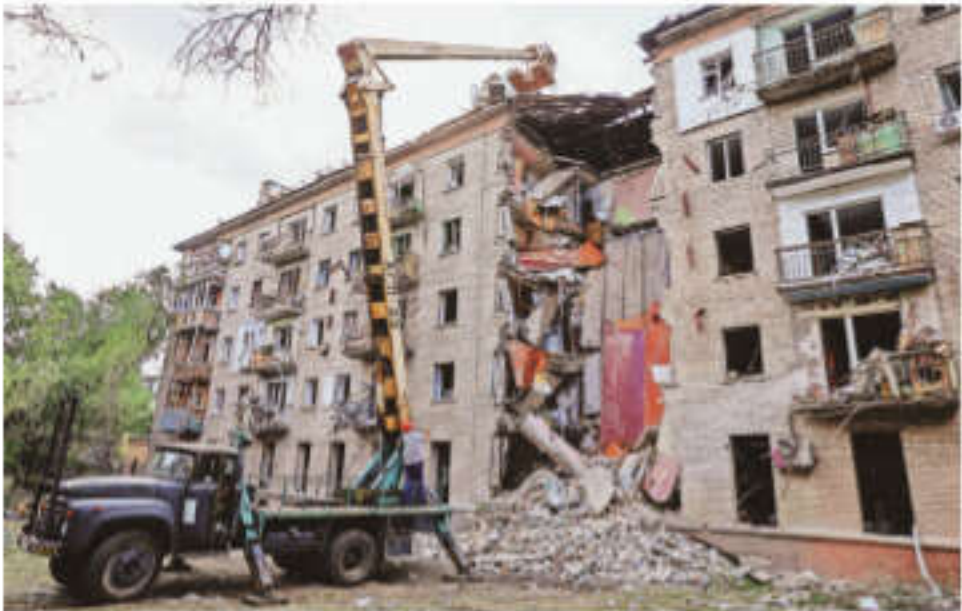
A residential building damaged in overnight Ukrainian shelling on Friday in Luhansk. Reuters
