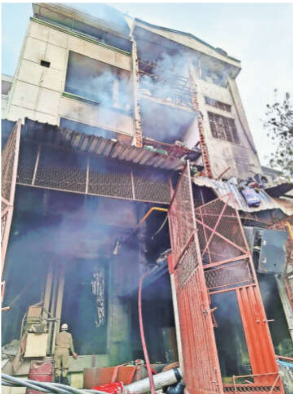
The four-storey factory, Shyam Kripa Foods Pvt Ltd, is located in the DSIIDC Industrial Area in Narela. PTI
