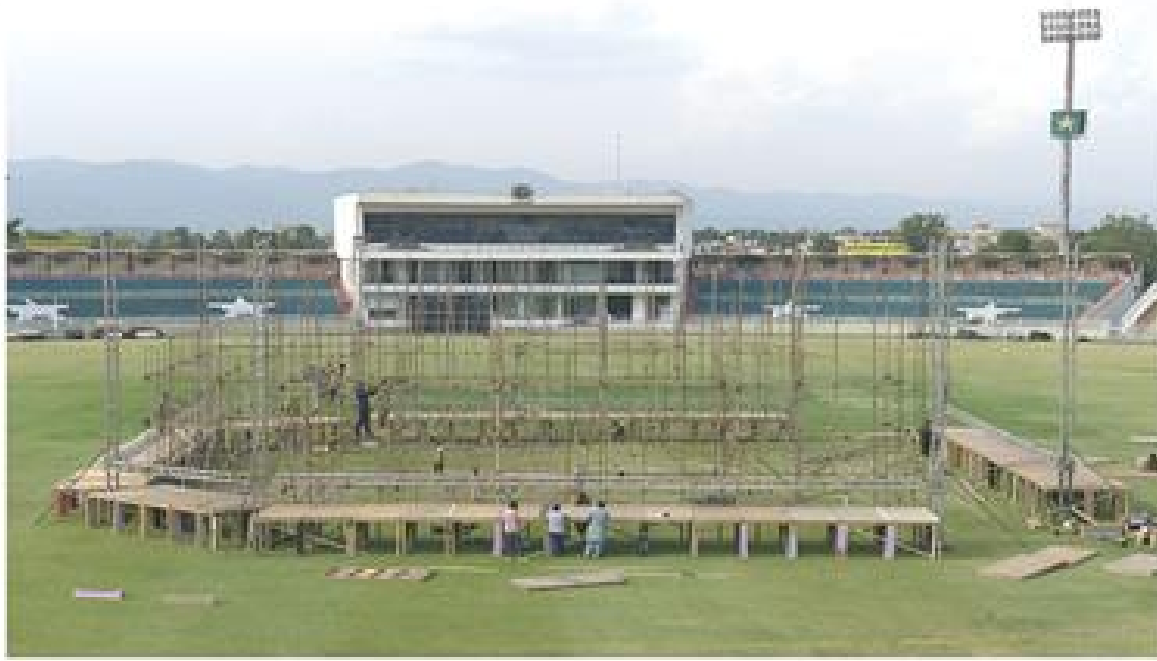
WORKERS build a structure to install a screen at the Rawalpindi Cricket Stadium on Friday where Pakistan-India match of the T20 World Cup will be telecast on Sunday (June 9). — Photo by Muhammad Asim
