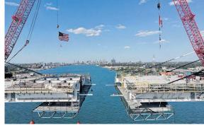
The gap between the bridge's Canadian and U.S. sides is seen in late May, with just 11 metres separating the span's two sides.
