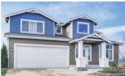
An Earthquake Soft Story (ESS) home with a living space built above the garage.
