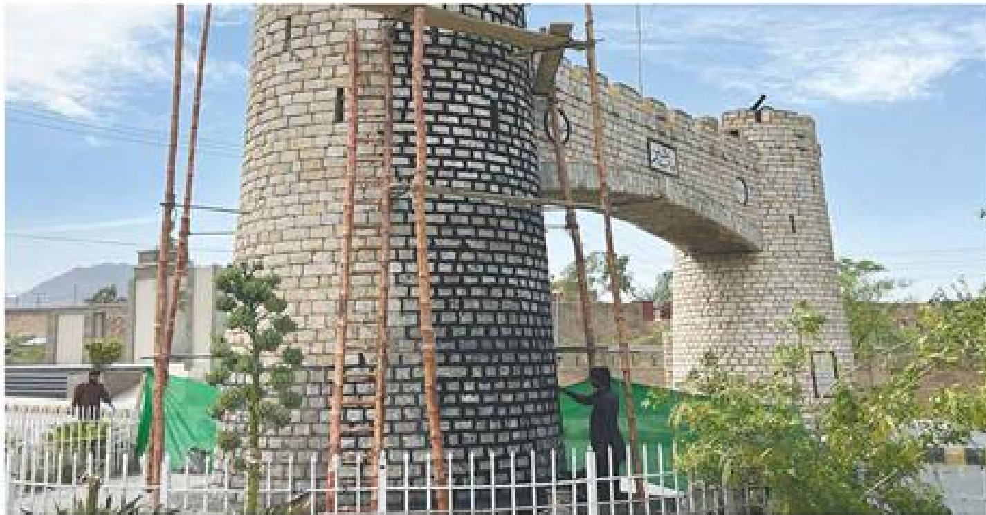
A MASON repairs Bab-ul-Khyber in Jarnud as part of a beautification plan. A gateway of historic Khyber Pass, it was built in 1904 by the then military ruler, Gen Ayub Khan. — Photo by Ibrahim Shihwarri
